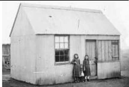
A corrugated iron cottage with shop counter on the goldfields (SLNSW Holtermann collection Digital Order No. a2823034)
