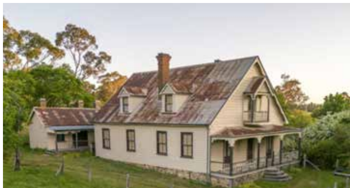
The exterior of Craigmoor House in Hill End Historic Site. Photo: John Spencer
